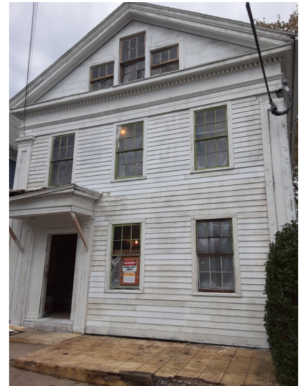
Original clapboard revealed
