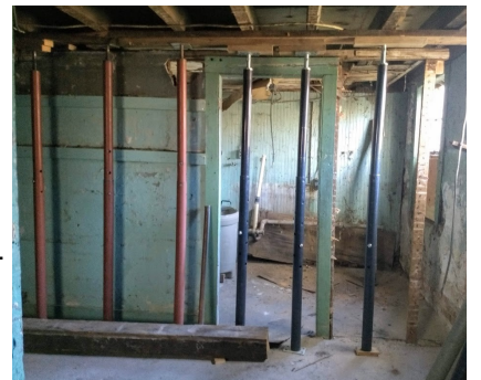
Jacking up a sagging floor
